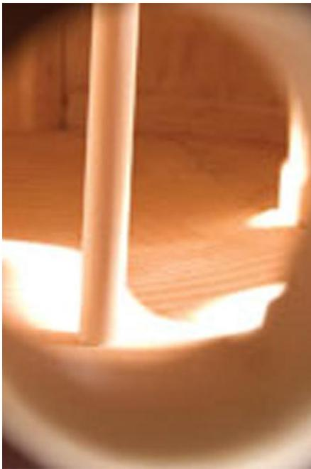
The post must stand straight and be cut to have full surface contact with both top and bottom plates.
